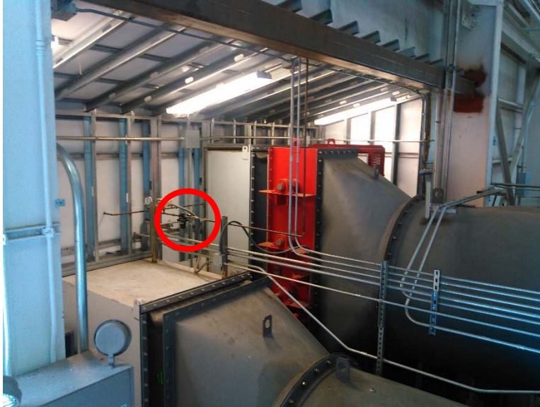
Figure 8 – Location of air pressure regulator
