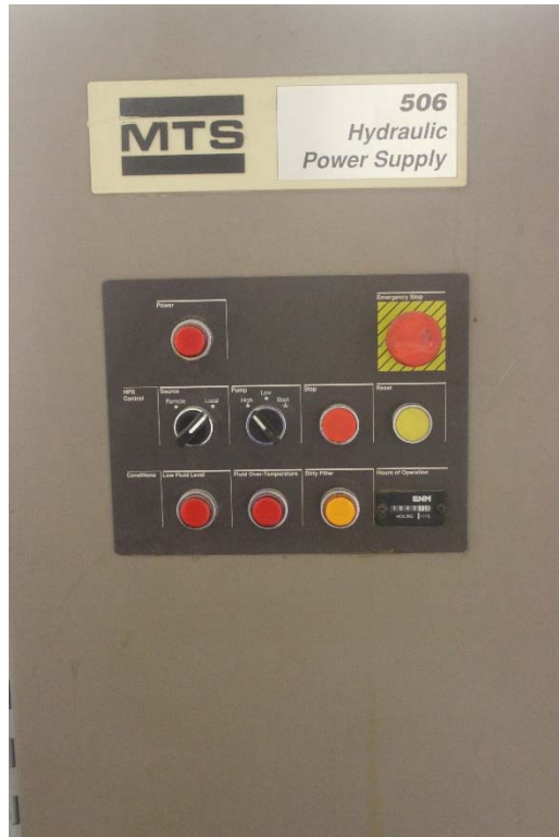
Figure 6 – HPU Control Panel
