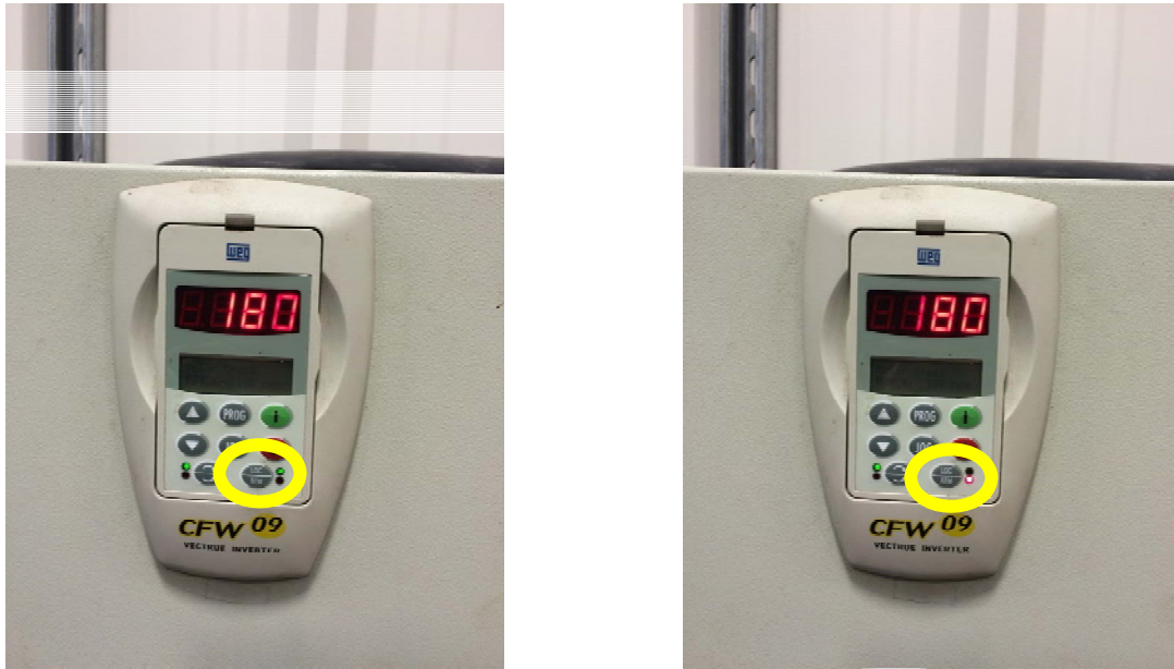
Figure 6 – Enacting remote functional capabilities of VFD
