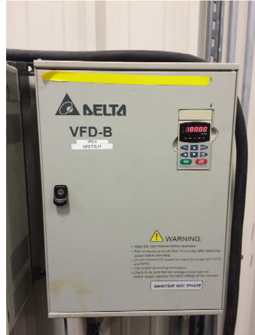
Figure 4 – Variable Frequency Drives (Blower #2 on left, Blower #1 on right)
